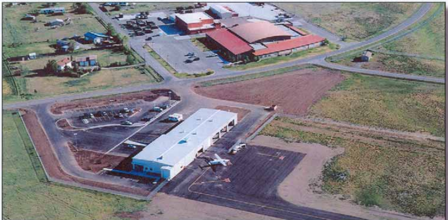
FedEx Facility at Gallatin Field - Constructed in 2005
